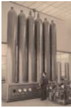
Accumulators for hydropneumatic plant 1940-1950
